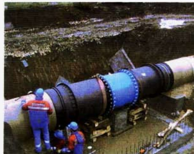
A Viking Johnson coupling being fitted to the Ruse water main
