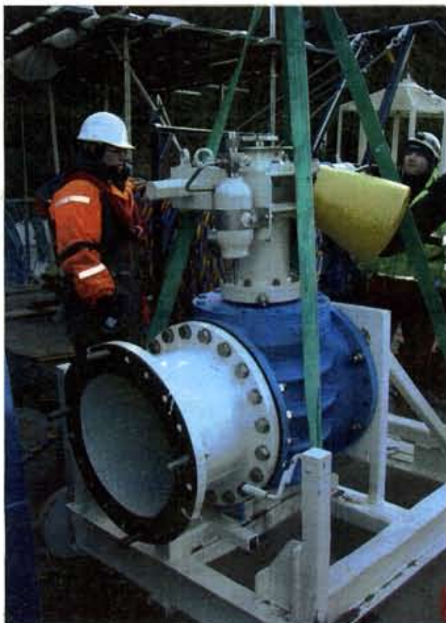
The Viking Johnson valve and trolley is lowered into the lake
