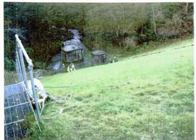
The pump house where the valve controls are situated
