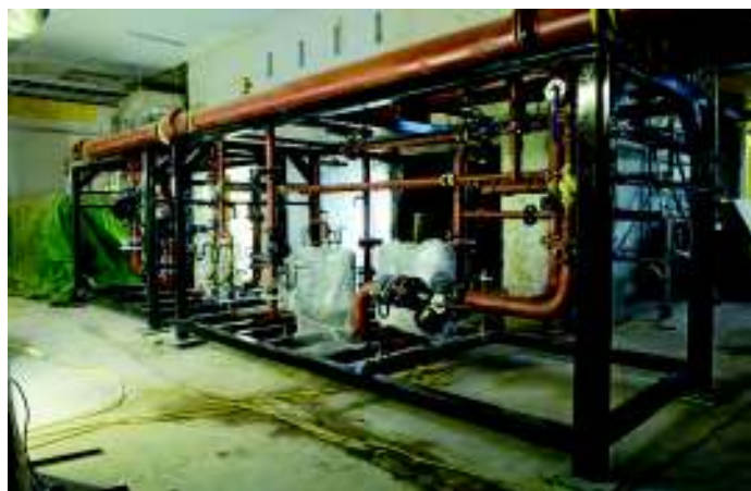
Crane Fluid Systems' valves installed within prefabricated modules, prior to installation in Rail House, Manchester.
