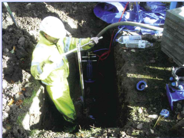
Viking Johnson Through Bore Hydrant and Hydrant Wizard in action
