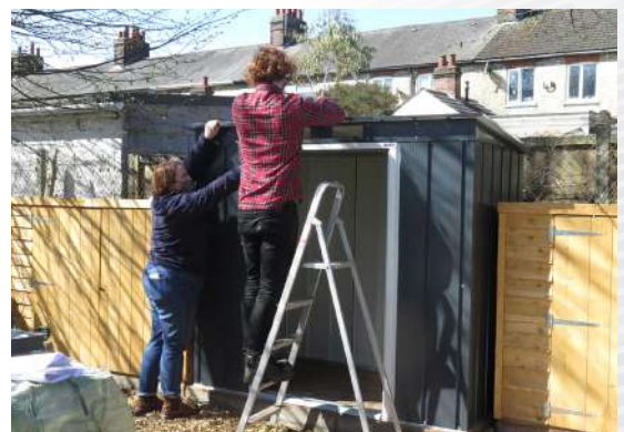
Crane Building Services & Utilities associates in Hitchin, UK, assembling a shed for Triangle Community Garden.
