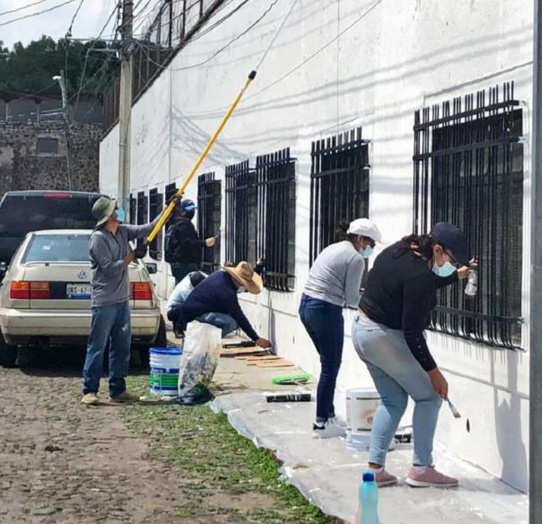
Crane Payment Innovations associates in Queretaro, Mexico, helping with building maintenance at the Centro de Protección de Ancianos.
