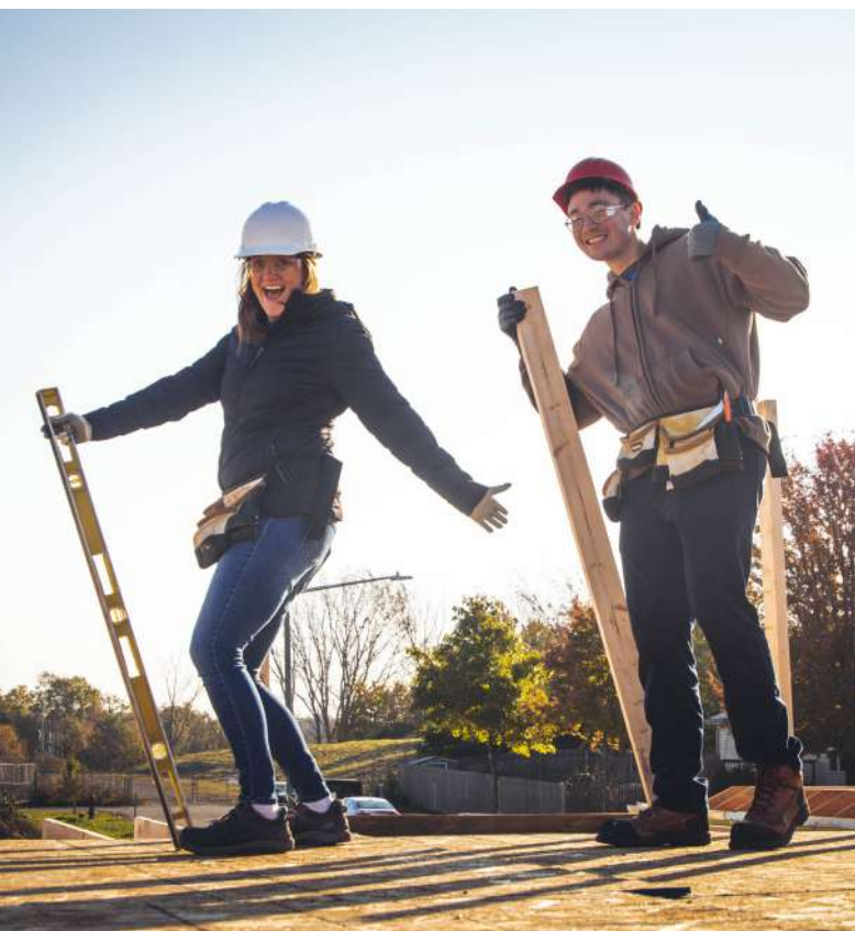
Crane Composites associates in Joliet, Illinois, working with Habitat for Humanity to build affordable housing.
