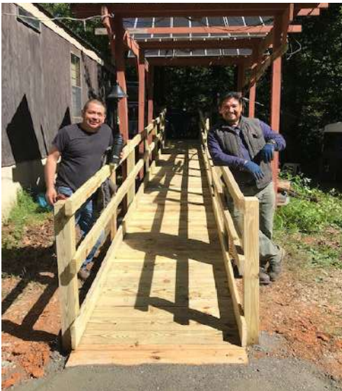
Crane ChemPharma & Energy associates based in Marion, North Carolina, building a wheelchair ramp as part of an effort by Pleasant Gardens Baptist Church to help the disabled in the area.
